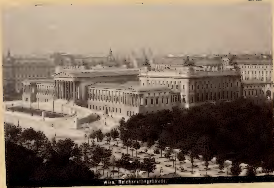
General View of Parliament House, Grecian Classical Renaissance - Hansen.
